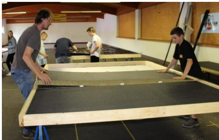
The insulation of the collector is important to prevent heat loss.
