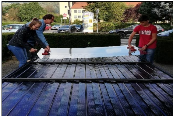
11. Cleaning and placing the glass on top on top
